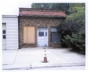
The south facade is red brick with the parapet stepping down toward the rear/east. The parapet has a tile coping. Irregularly-spaced windows are the original 12-light steel units with operable 6-light panels. The rear facade shows evidence of former patching on each side of a central oversized door with an overhead garage door in place. There is significant spalling of brick and open mortar joints on the rear facade. A square brick chimney rises above the roofline at the northeast corner.
