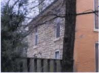
KDOT/Blackwell photo 2, south side of home showing the limestone wall with cut limestone lintels and sills, vinyl storm window has been added. 2015
