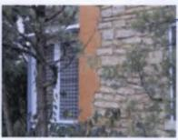
KDOT/Blackwell photo 7, close up of northeast corner showing the stone work and some brick work under stucco. 2015
