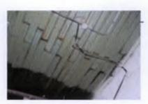
127 S. Kansas Ave. Deteriorated fluted beadboard ceiling on 1st floor. Spencer. 09/12/2014
