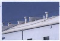
631 SW 1st. Detail of membrane roof wrapped over south parapet, looking SW from east side. Spencer, 03-06-2015.
