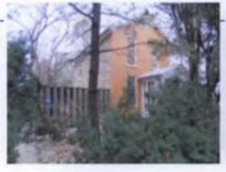
KDOT/Blackwell photo 1, southeast corner of house with painted brick facade and limestone wall with cut limestone lintels and sills. 2015
