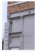
127 S. Kansas Ave. Cast-iron column at street entry to 2nd floor on front facade. Spencer. 09/12/2014
