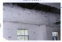
124 S. Harrison. Interior detail of block & brick wall, fiberboard ceiling and steel window. Spencer. 09/17/2014
